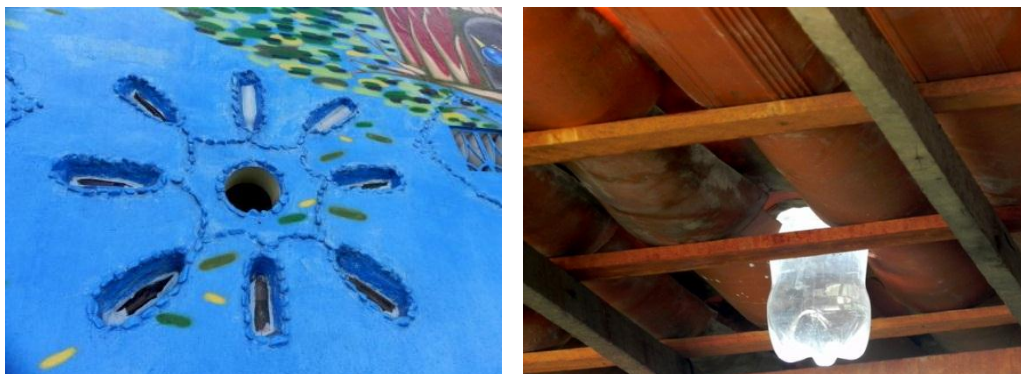
Figure 3. Examples of natural illumination at Escola Vila using both glass and plastic bottles. Source: this research.
