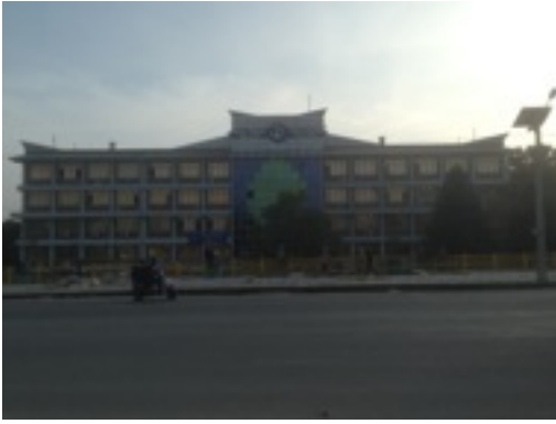
Image 1.3 Nepal Telecom Headquarters
