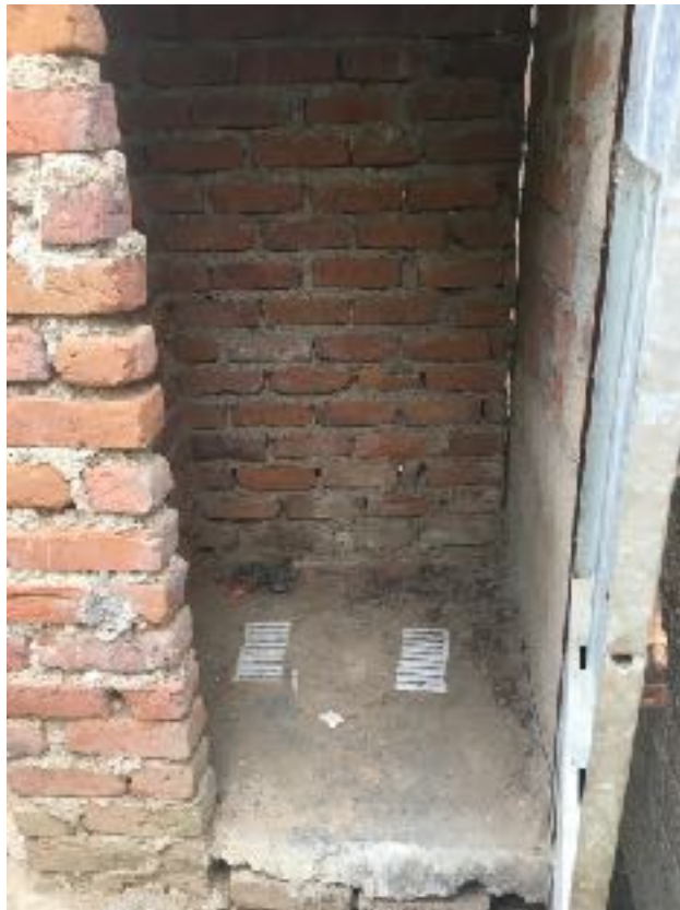
Figure 8: A government-constructed latrine in Umarni Village with no pit.
