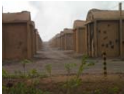
Lines of industrial coal ovens
