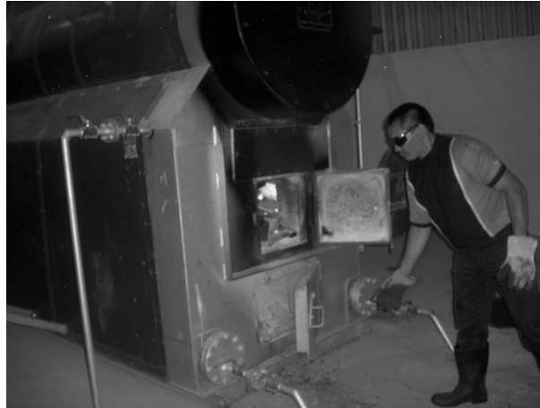
Figure 1: Wood being added to the boiler in the biomass power plant.
