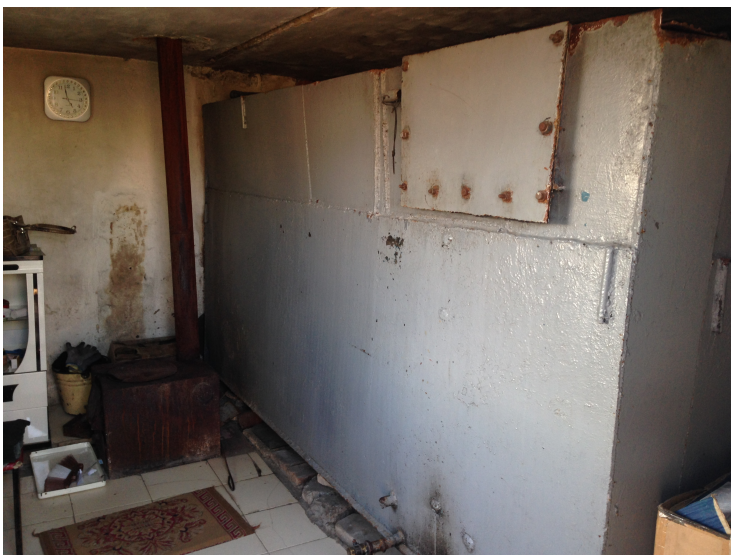
Figure 4: The inside of a kiosk that distributes water via tank. To the left is the small stove, meant to keep the kiosk warm.
