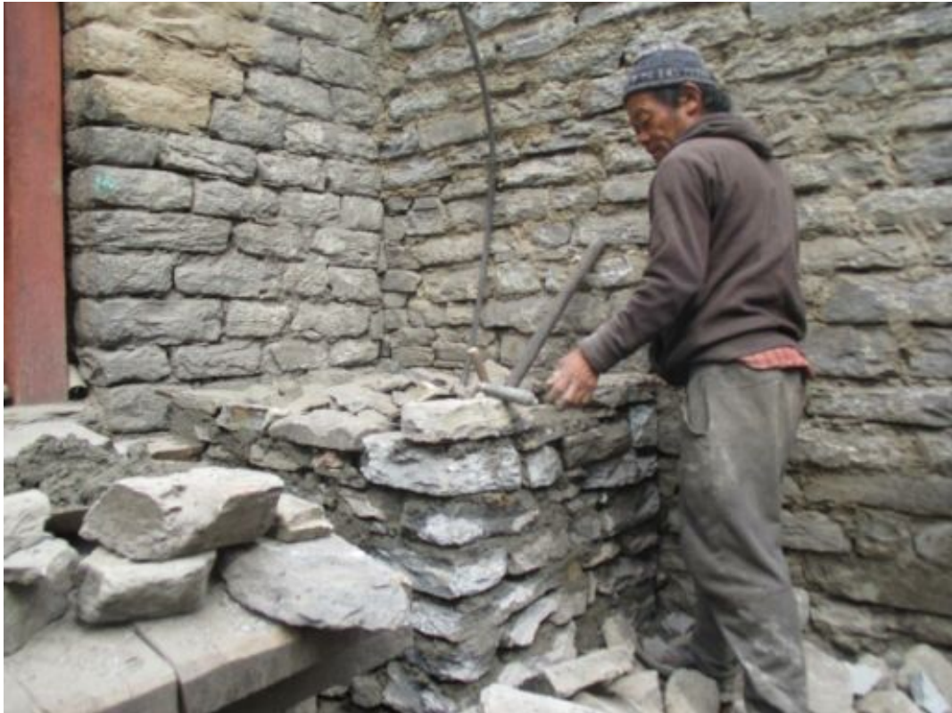
Picture 7: A villager repairing a village house
