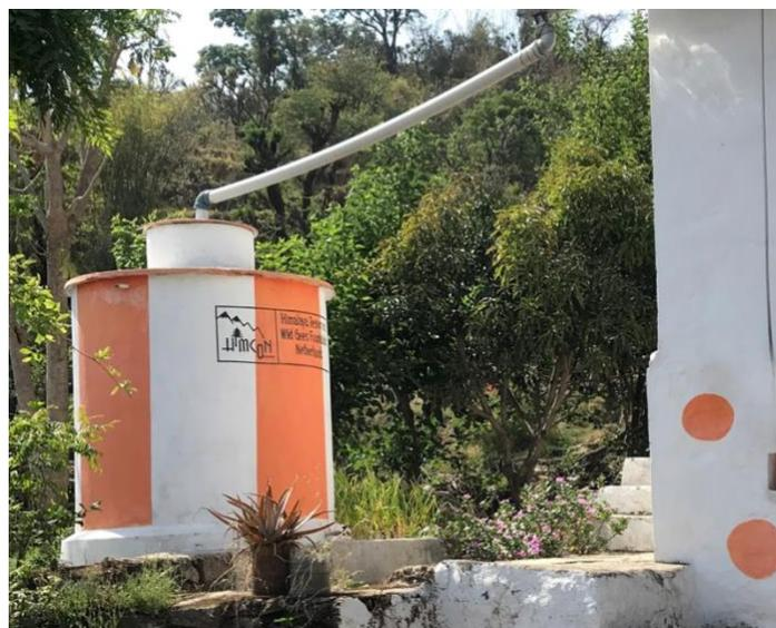
Image 5: A decoratively painted HIMCON water storage tank in a village home. The tank is constructed from low-cost Ferro-cement and can hold up to 5000 litres of water. This tank has a pipe connected to it for harvesting rainwater from the roof (Author).
