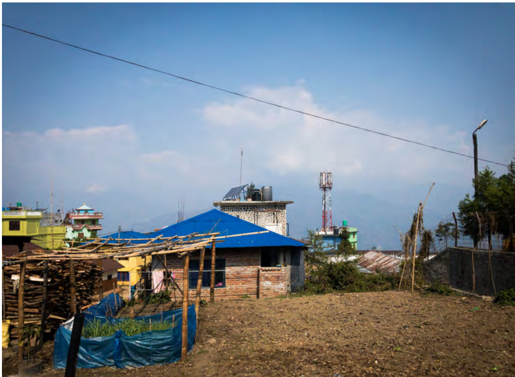
View of the NTC office and its's signal pole on the top of the building from a distance in Taplejung
