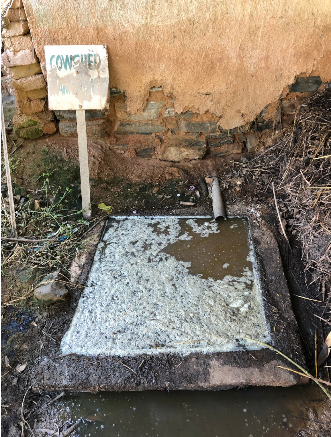
Figure 3. Cowshed management: Urine drainage system
