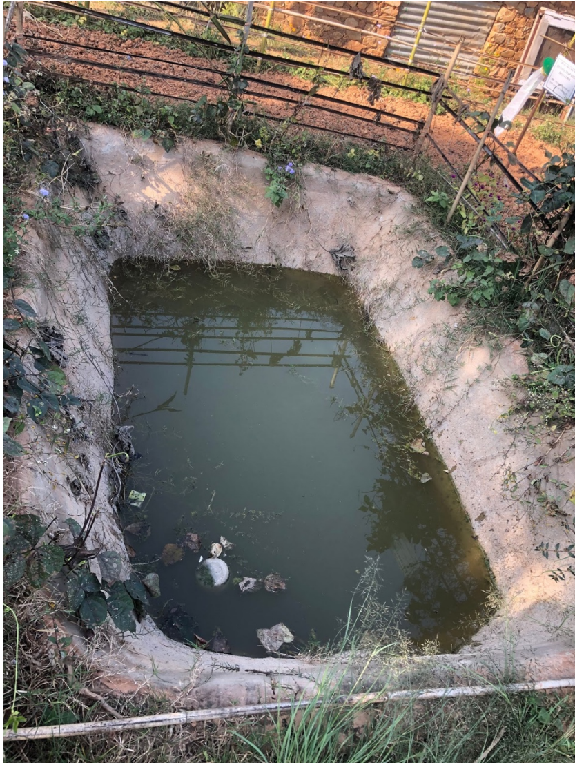
Figure 1. Soil cement tank
