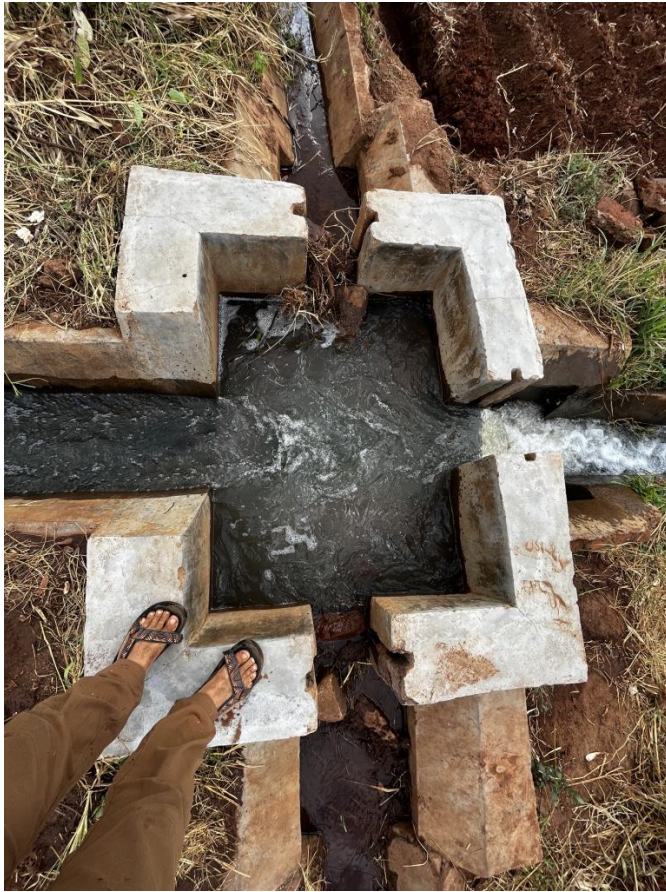
Figure 6: A concreted block distribution box in the lower section of the scheme. Block A faces right (east) and Black B faces left (west).
