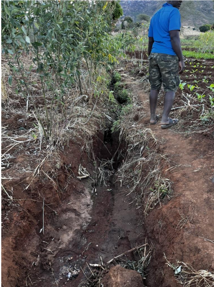
Figure 11: Deep soil-erosion occurring in the un-concreted lower section of the main canal at Kamwaza Irrigation Scheme.
