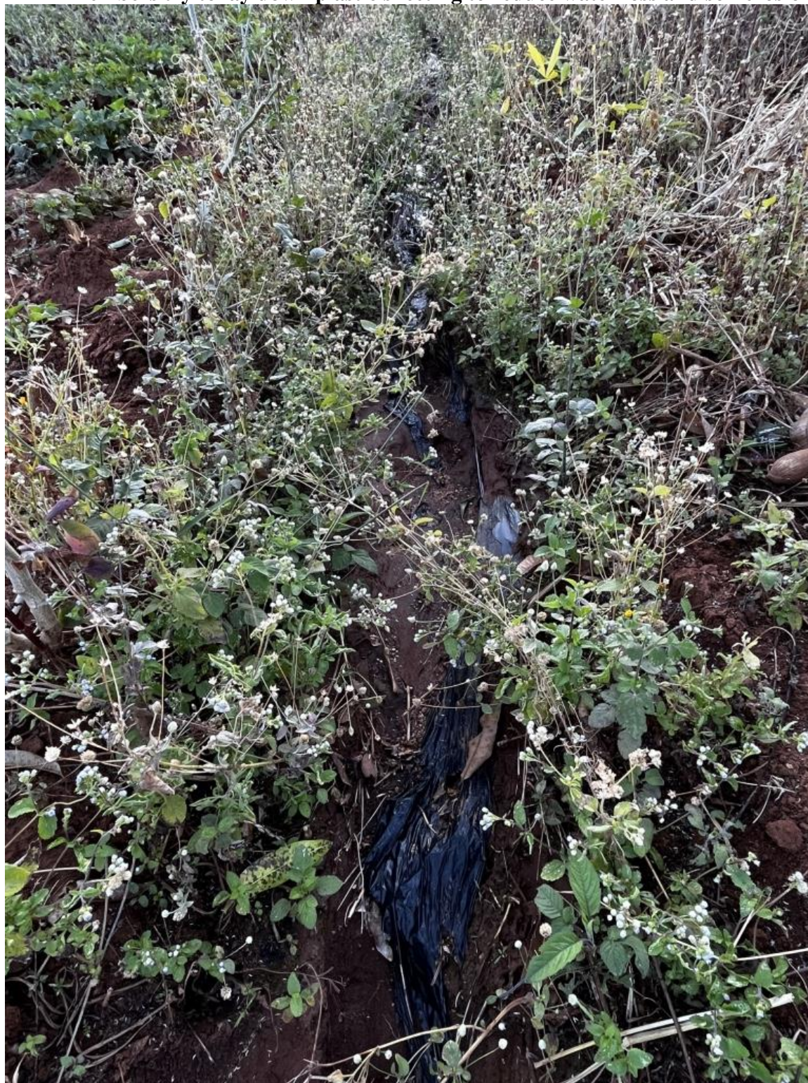
Appendix T – A section of the non-concreted main canal at Kamwaza Irrigation Scheme. Members try to lay down plastic sheeting to reduce water loss and soil erosion.
