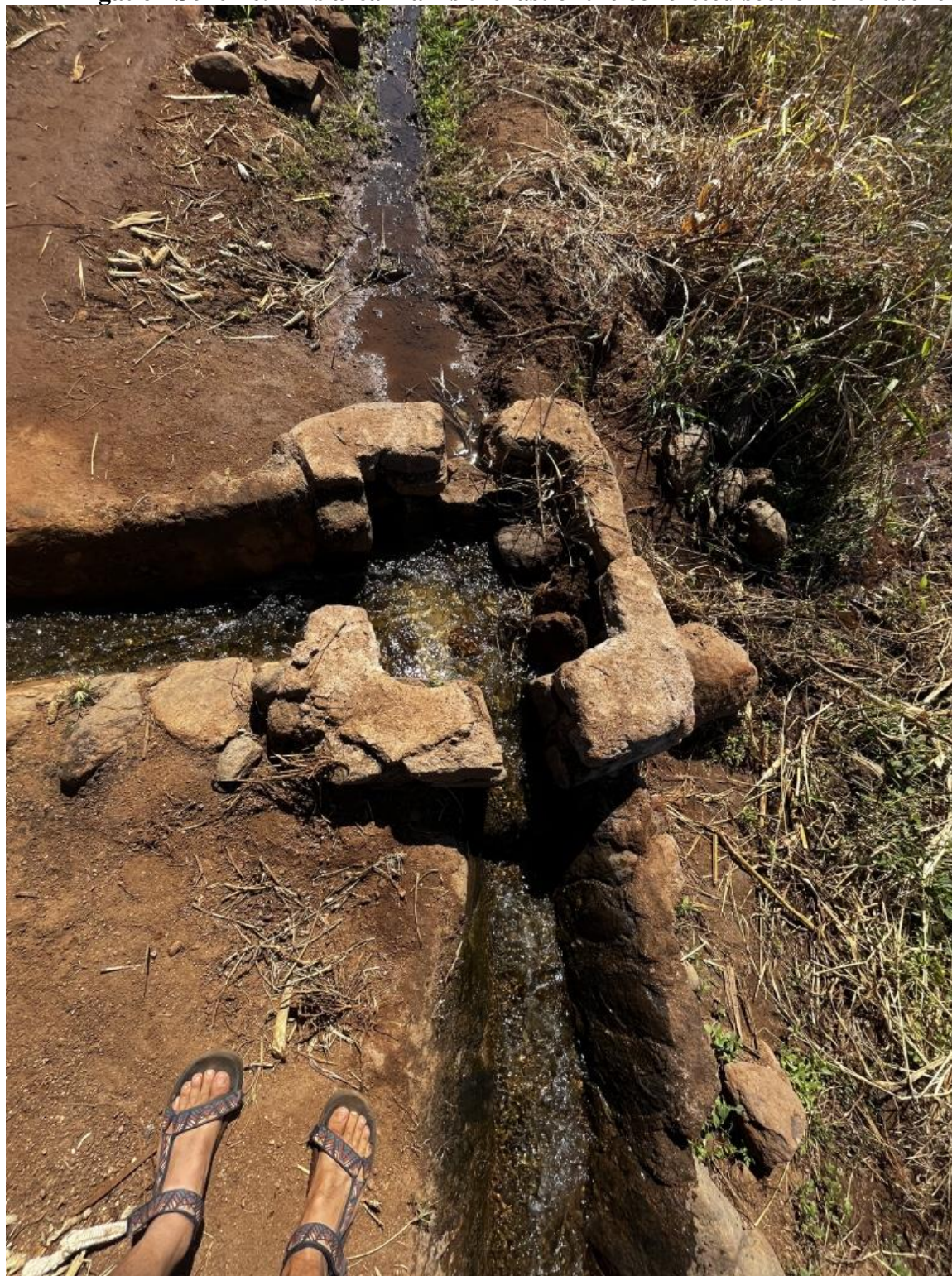
Appendix S – The final concreted distribution box in the middle section of the Kamwaza Irrigation Scheme. This area marks the last of the concreted section of the scheme.
