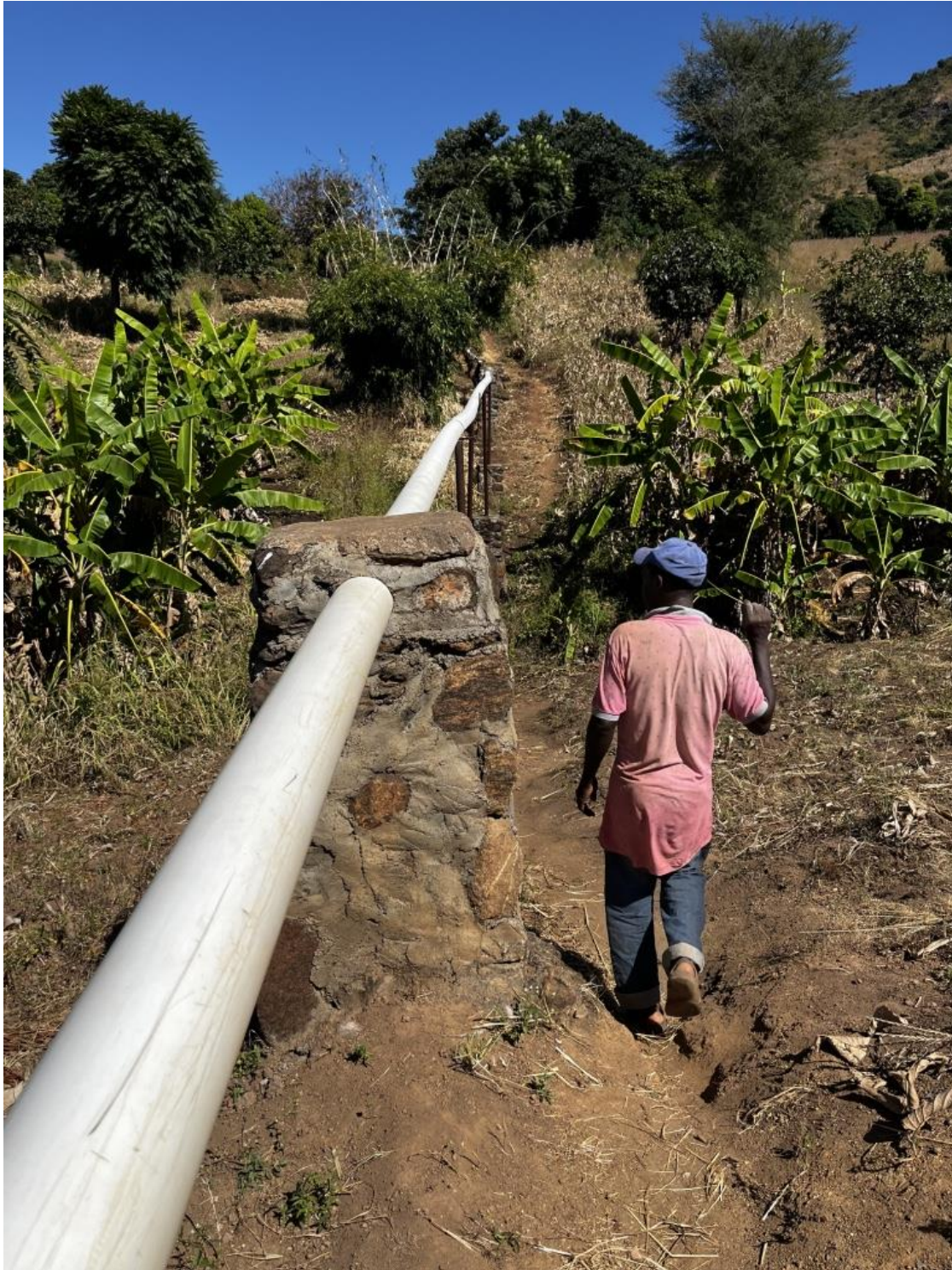
Appendix O – Jameson Viah (Secretary) displays concrete slabs securing pipes transferring water across a sloped valley in the upper section of the Kamwaza Irrigation Scheme. Built in 2014 with NGO, CARE Malawi. Banana trees border a small river crossing.
