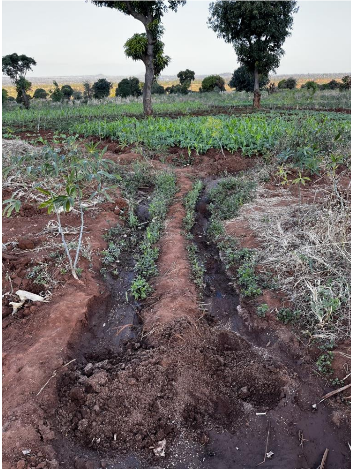
Figure (10): A photograph of the non-concreted portion in the lower half of Kamwaza irrigation scheme.
