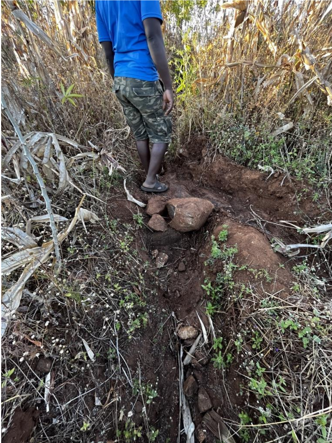
Appendix U – A distribution intersection held together by rocks and soil of the non-concreted section of the main canal at Kamwaza Irrigation Scheme. Tall, dry maize stocks surround the canal.
