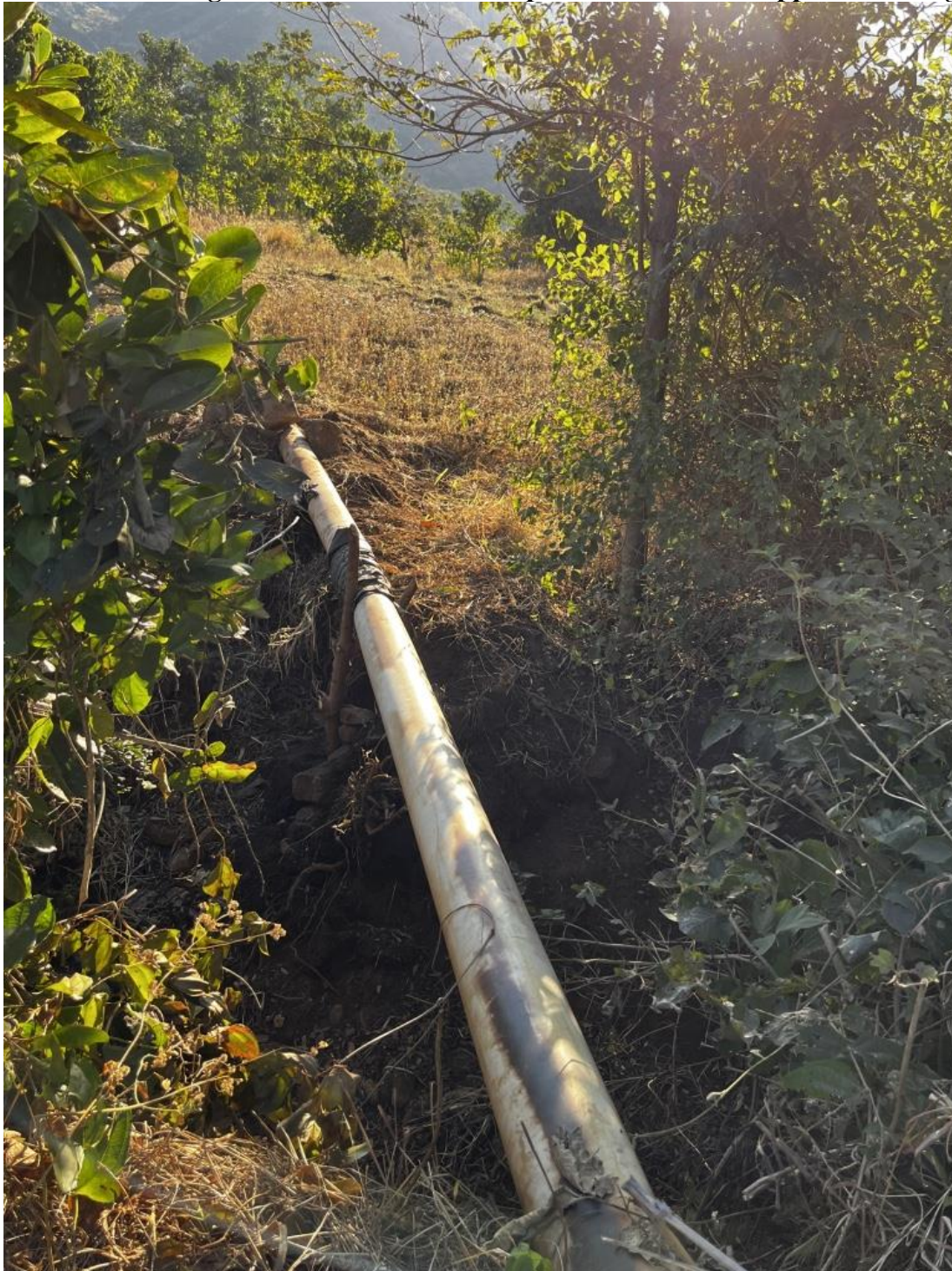
Appendix K – A maintained water distribution pipe located on the southern border of Chauluka Irrigation Scheme. Plastic wrap and local timber support the bridged pipe.
