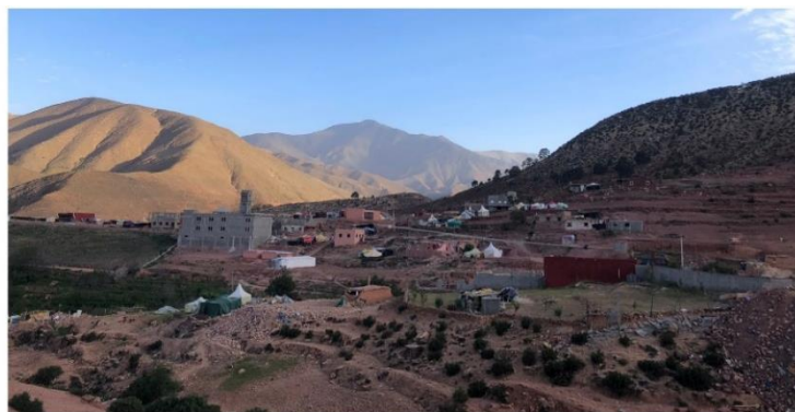
Figure 3.1. Inghede partial destruction and severe damage
