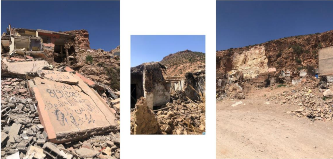
Figure 7.1. Imi n Tala and Adrouz villages 7 months after the earthquake
